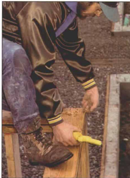
Blocks make sure the line stays straight. A traditional method of lining is to nail blocks at each corner and to string line across the blocks. Blocks hold line away from the plate. Another block gauges distance between string and plate.
