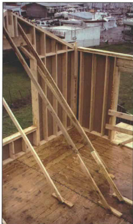
Line braces hold walls straight. This gable end is straightened and held straight with 2x4 line braces. Note the line running along the blocking. The top of each brace is nailed to the wall just below the plate. The bottom of each brace is left square so that it can be pushed forward with a crowbar, just like a racking brace. When the wall is straight, the line braces are nailed to cleats. The cleats are spiked to the floor joists, not just to the plywood deck.
