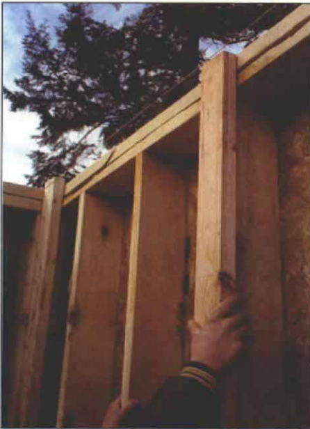
Blocks make sure the line stays straight. A traditional method of lining is to nail blocks at each corner and to string line across the blocks. Blocks hold line away from the plate. Another block gauges distance between string and plate.
